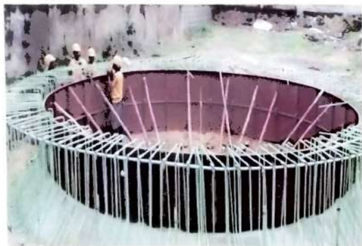
CONSTRUCTION OF SUCTION WELL AT SM NARAYANAN NAGAR
