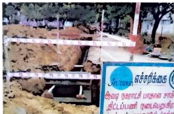
PACKAGE - II THIRUKKURAL STREET (LAYING 600 MM DIA DI PIPE)
