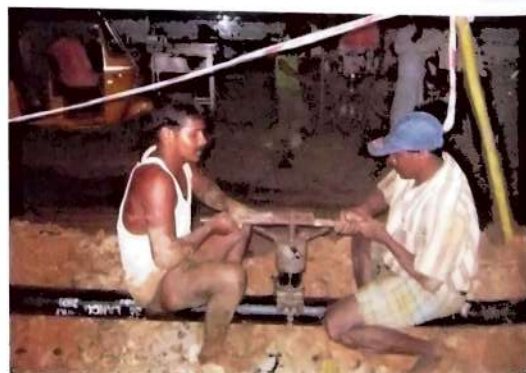
RENEWAL OF HOUSE SERVICE CONNECTION WORKS UNDER LEAK DETECTION & RECTIFICATION
