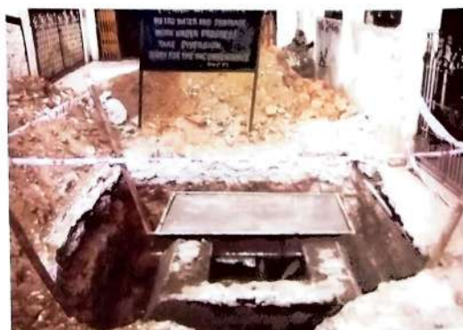
MANHOLE CONSTRUCTION AT EVR STREET
