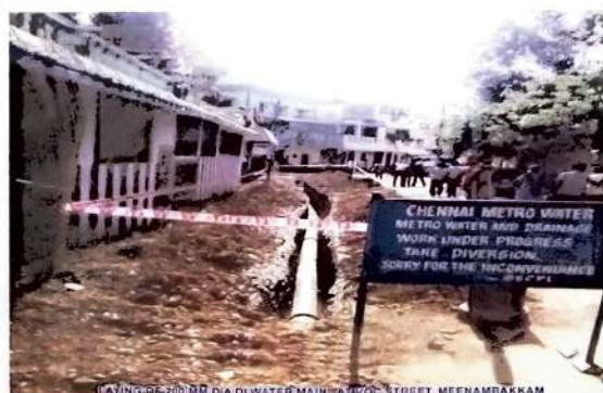
LAYING OF 200 MM DIA DI WATER MAIN AT VOC STREET, MEENAMBAKKAM
