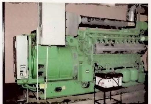
KODUNGAIYUR 110 MLD STP - BIO GAS ENGINE
