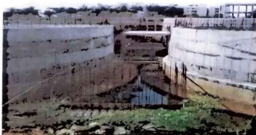
DIVIDING CHAMBER RAFT COMPLETED WALL REINFORCEMENT WORK UNDER PROGRESS
