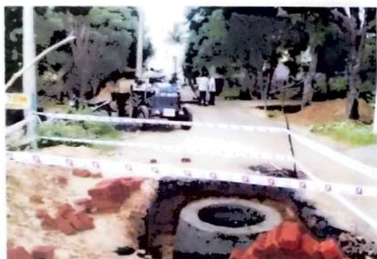
CONSTRUCTION OF MANHOLE
