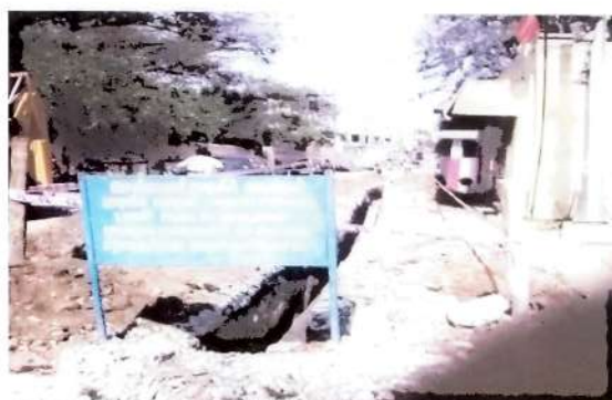
LAYING OF 200 MM DIA DI WATER MAIN AT KAMARAJ STREET, MEENAMBAKKAM
