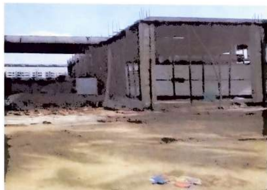
AIR BLOWER, MCC, HT SUB STATION, TRANSFORMER & DG BUILDINGS COLUMN COMPLETED UP TO ROOF SLAB
