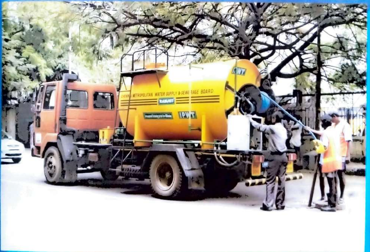
JET RODDING MACHINE OPERATION IN AREAS
